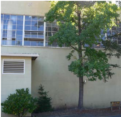
Campus central heat plant.
