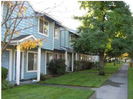
Housing for students with families is complementary in scale and design with adjacent residential neighborhoods.
