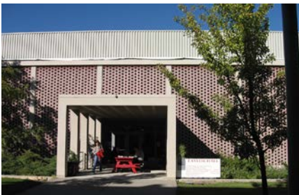
The unfortunate shading strategy employed at Taylor Hall disconnects building interiors and the landscape, creating a sense of ‘deadness’ around the building, and limiting daylight inside.
